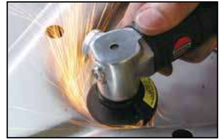
▲ Operation of Cutting Metal Plate
