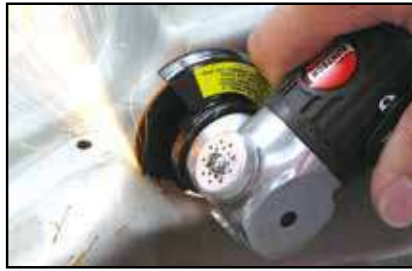
▲ Operation of Cutting Metal Plate
